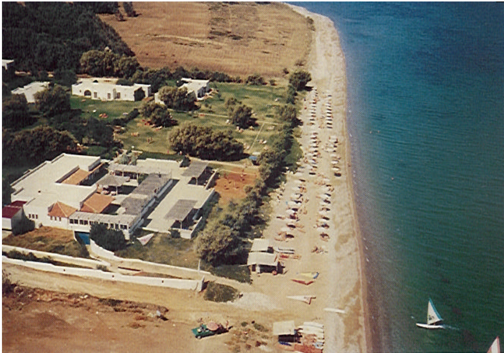
Shoreline before breakwaters system construction
