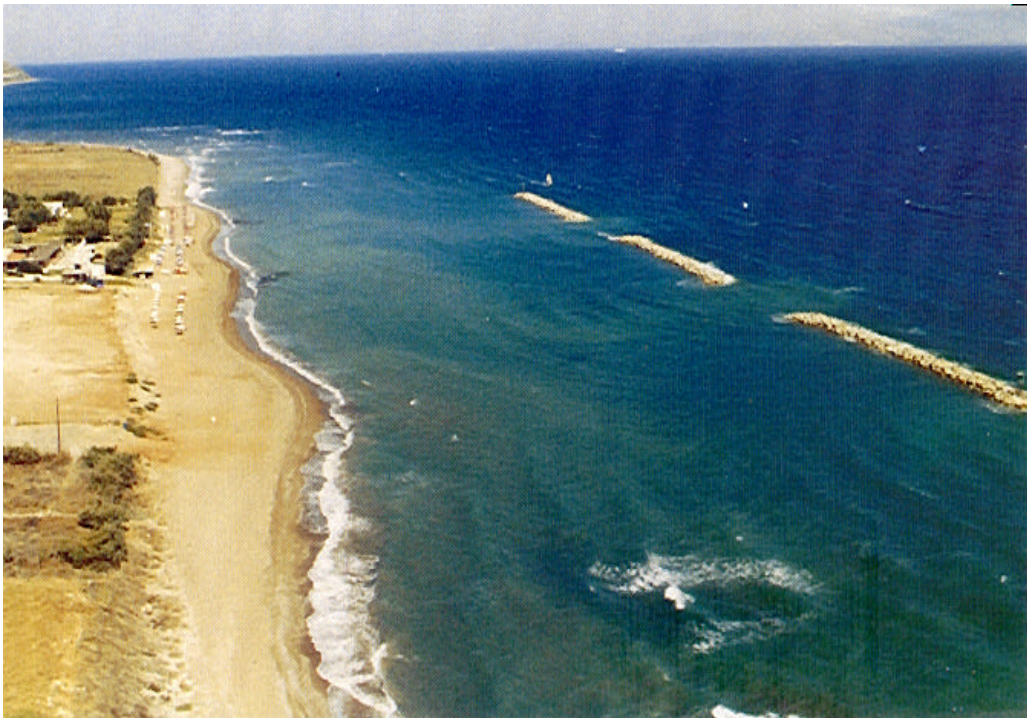
Shoreline after (1 year) breakwaters system construction
