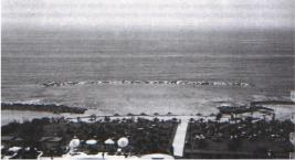
No. 003 consists of tree successive detached breakwaters parallel to the shoreline. The scheme was constructed in 1992 in order to protect and stabilize a 300 m sandy beach section that lies in front of a hotel. The beach was particularly vulnerable to wave attack which posed hazards to the swimmers.
